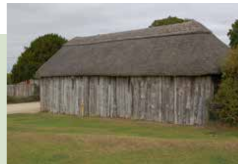
White Cottage barn Woodgreen 18th century 4 bay barn with split trunk walling and thatched roof
