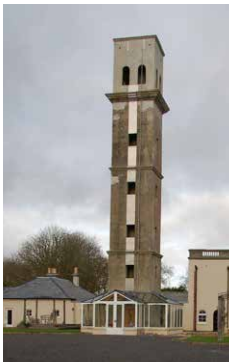
Trial tower c.1880 for ATT Peterson, early example of concrete construction
