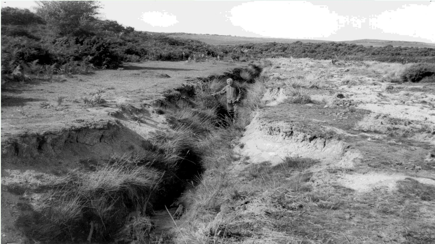
Aug. 1980. Drainage ditch eroded and enlarged by storms. An example of drainage NOT undertaken with "DUE REGARD TO THE INTERESTS OF AMENITY" (1949 Act)
