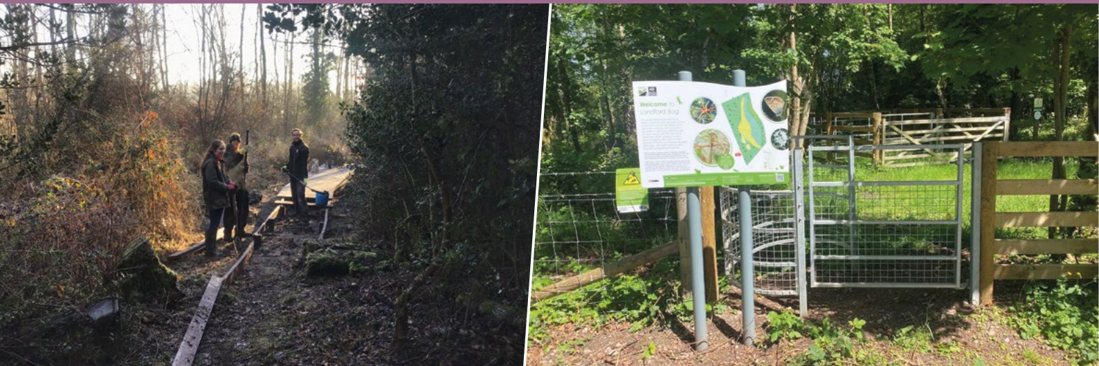
Left: Installing a boardwalk, and right: a new kissing gate and signage to improve access at Landford Bog
