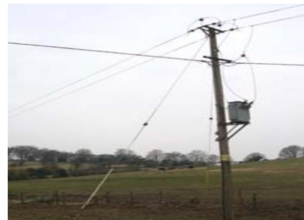
Overhead wires Blissford
