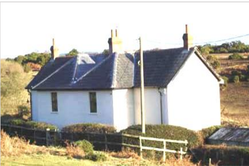
Extension reflecting the main building
