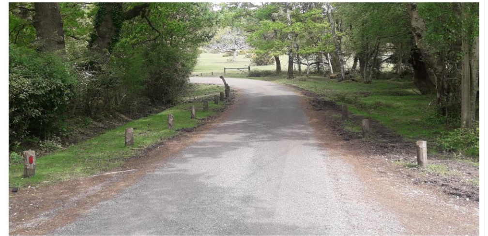
Verge restoration, before and after.
