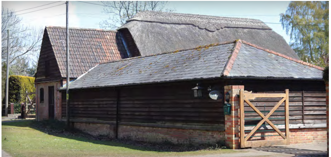
Traditional weatherboarding and roofing materials on agricultural buildings in Burley
