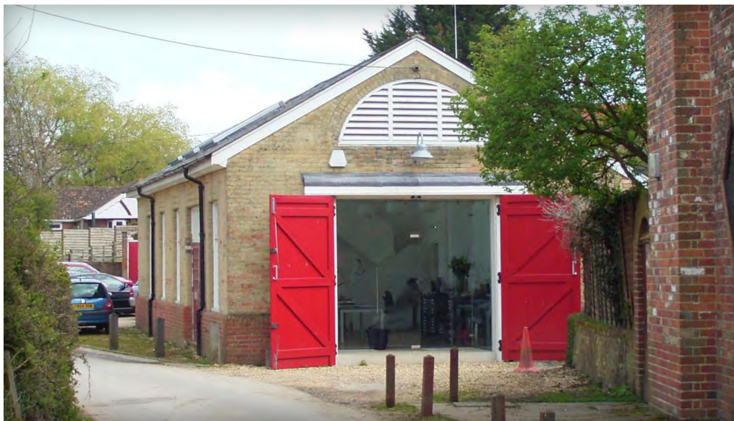
The successful conversion of the former Fire Station at Beaulieu into a design studio, which has retained the simple robust form and utilised existing openings
