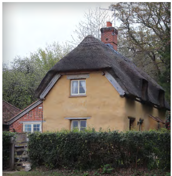
A cottage in Woodgreen rebuilt in cob after fire damage
