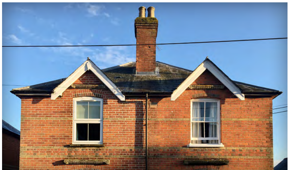
A pair of cottages showing the difference in frame size, finesse and detailing between UPVC and timber frames
