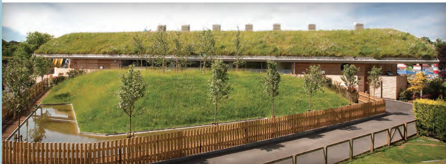
The successful use of a green roof at Paultons Park theme park
