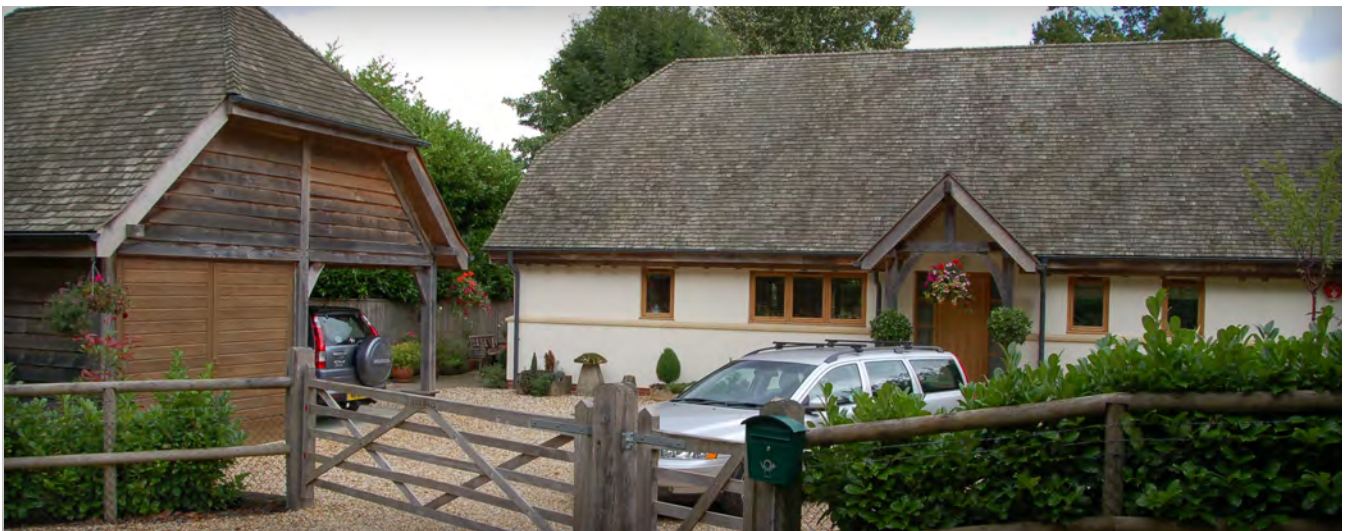
A shingle roof on a new build cottage in Burley
