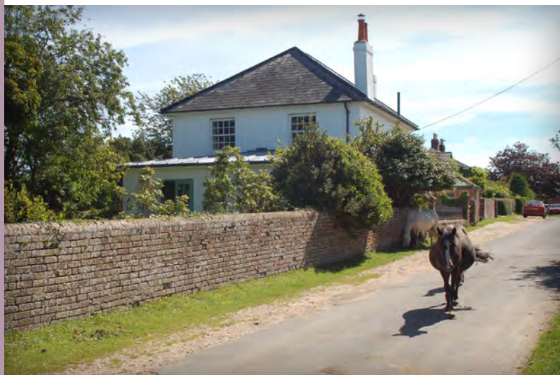
A typical low brick wall boundary behind a soft grass verge
