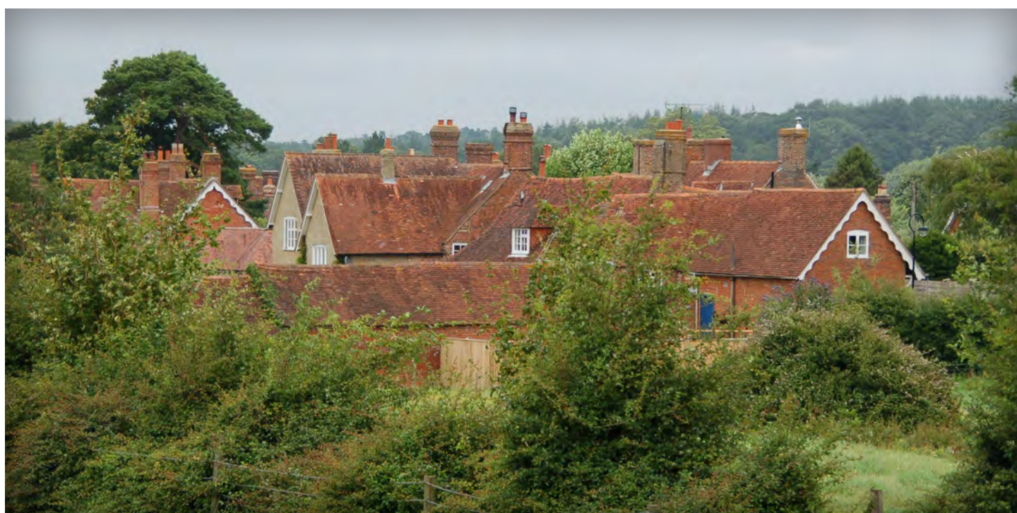
The rhythm of clay roof tiles, chimneys and steeply pitched roofs in Beaulieu
