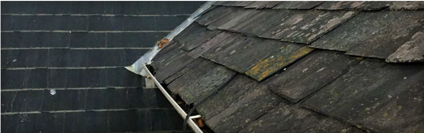
A photograph showing traditional natural slates (right) next to modern shiny slates (left)
