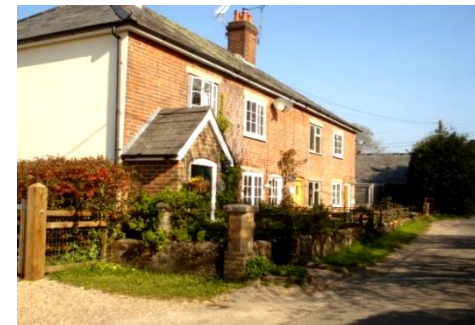
Terraced cottages Stuckton Hill
