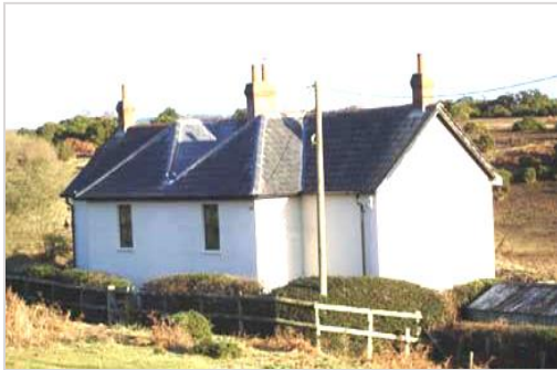
Extension reflecting the main building
