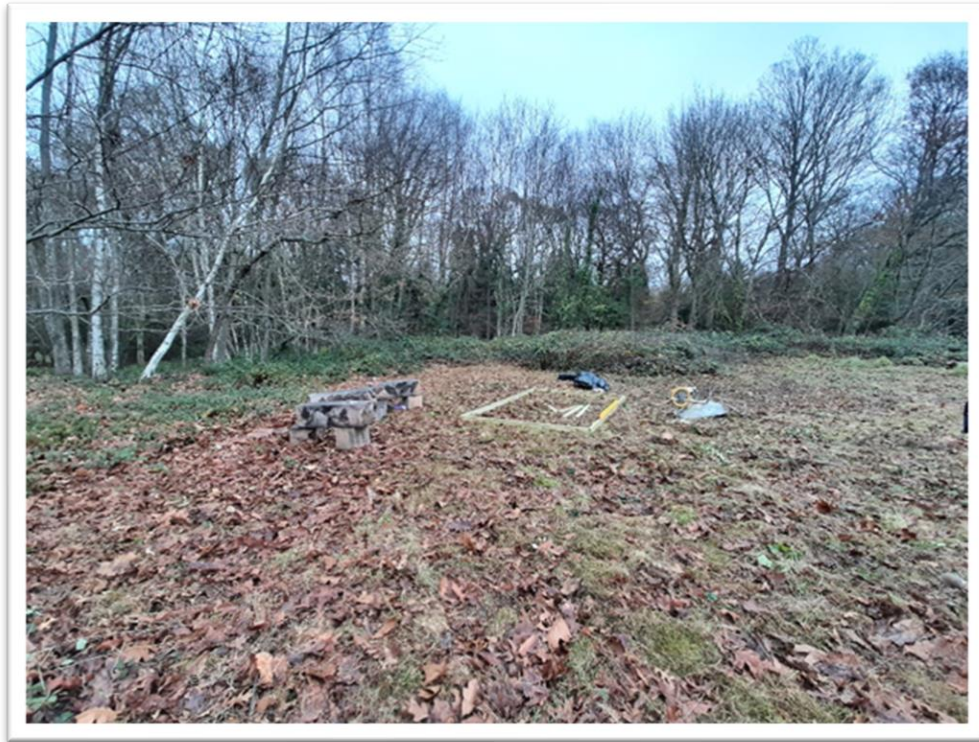
Insulation of carved bench underway, Dec 2021
