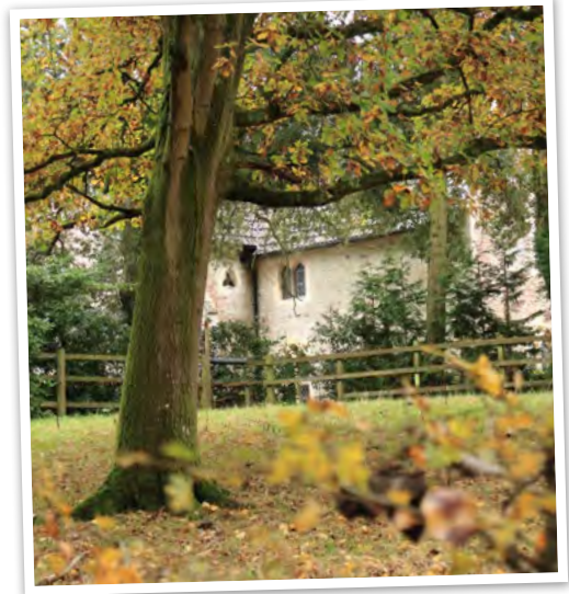
View from the trail of Dunclagh with its mullioned windows with Bath Stone.
