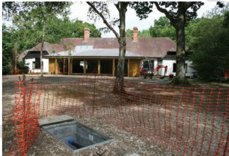
Ground source heat pump installation at Ferny Crofts Scout Activity Centre, near Beaulieu
