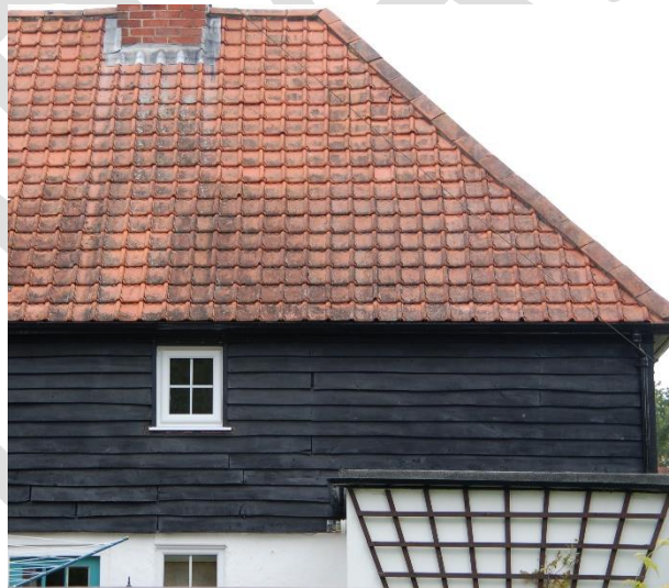
Pantiles and Bridgewater tiles are common on Arts and Crafts properties in Lyndhurst and Burley
