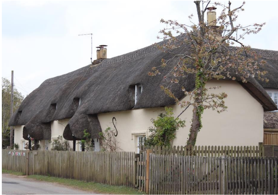
A pair of lime plastered cob cottages under a thatched roof with a traditional simple flush ridge, in Hale
