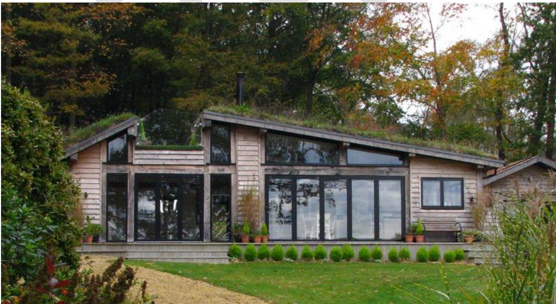
A modern development in Woodgreen that has successfully used a green roof, structural glazing, and careful massing to nestle into the landscape
