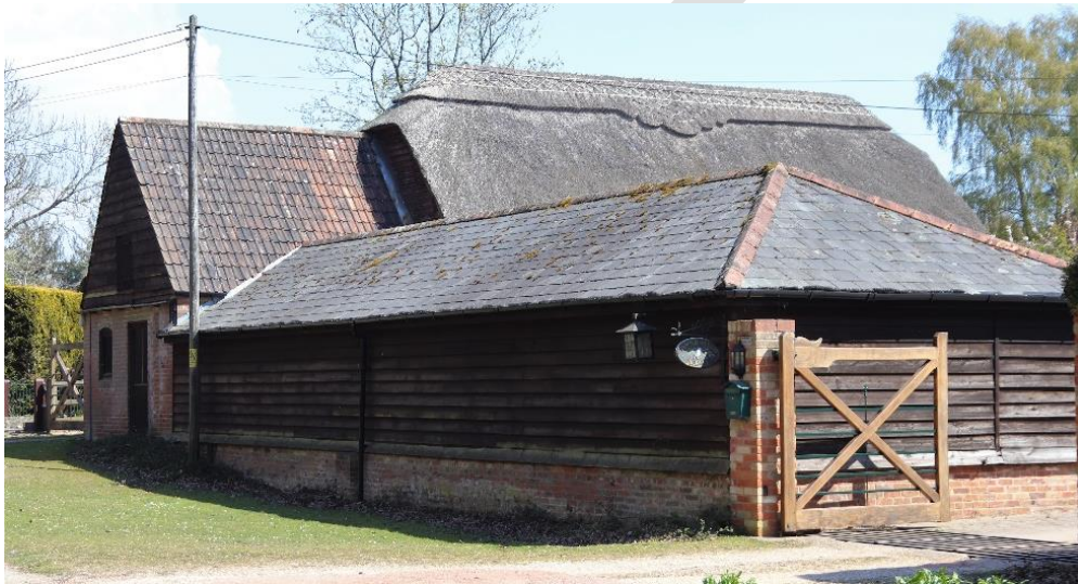
Traditionally weatherboarding on an agricultural outbuilding in Burley
