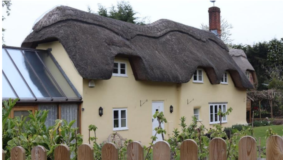
An example of a small commoners dwelling that has been extended over time
