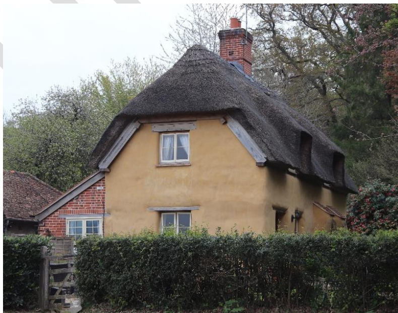
A cottage in Woodgreen rebuilt in cob after fire damage
