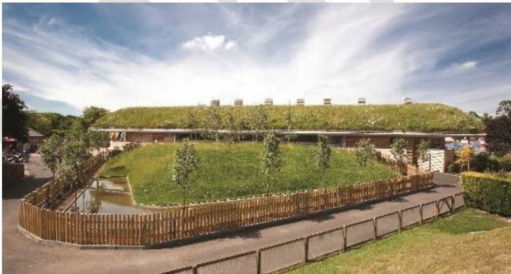
The successful use of a green roof at Paultons Park theme park
