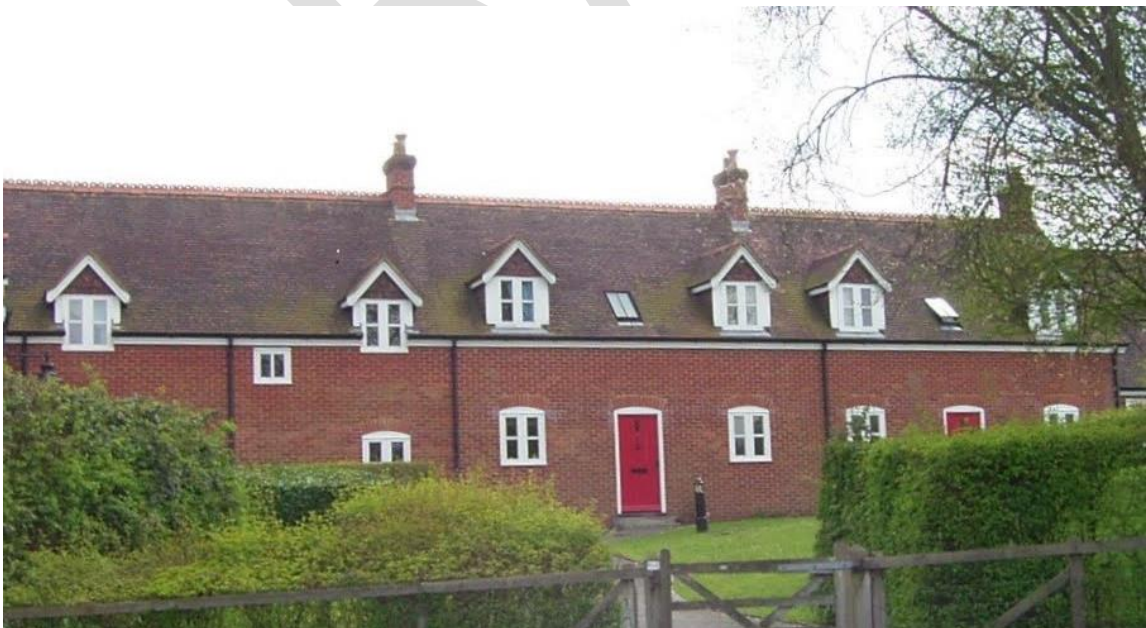
Cottages at Beaulieu with small roof dormers and discrete rooflights
