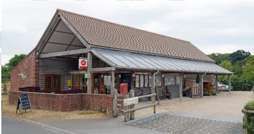
Woodgreen Community Shop with integral solar panels on the south-facing canopy
