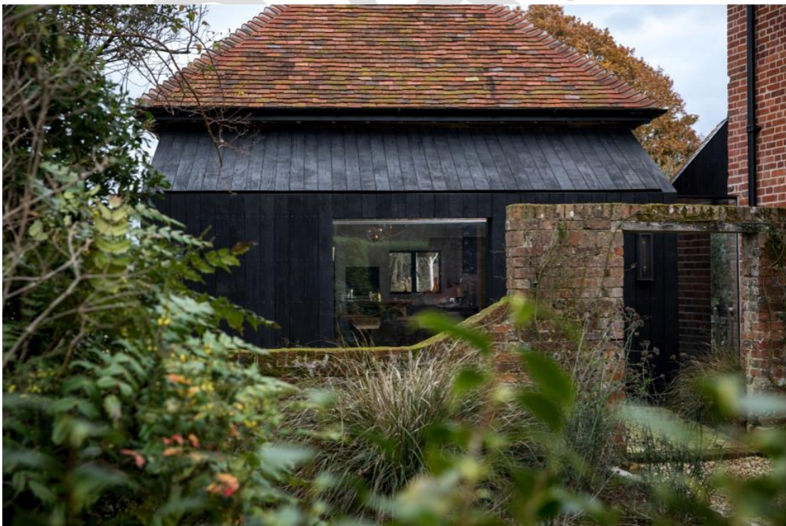
A successfully designed partially glazed & timber link between a farmhouse and the adjacent barn near Exbury
