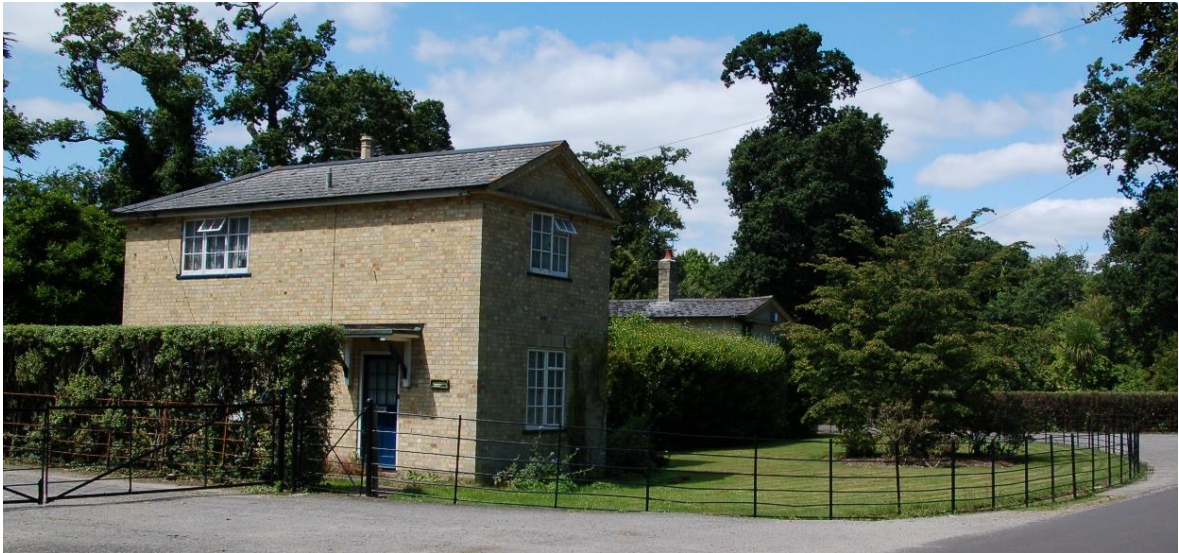
Traditional estate railings around the Exbury Estate lodges
