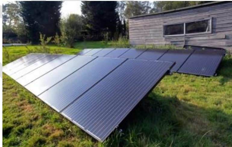
Ground mounted solar panels at Efford Mill
