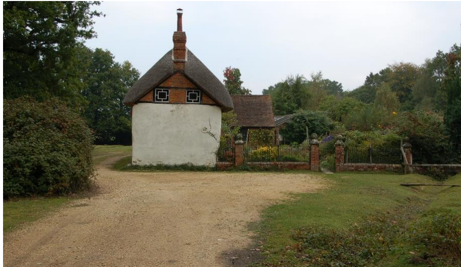
A simple informal gravel accessway and a boundary ditch
