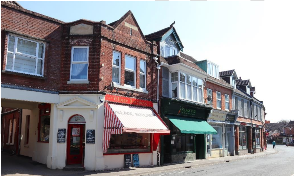
Higher density, varied development along Brookley Road in the village centre of Brockenhurst
