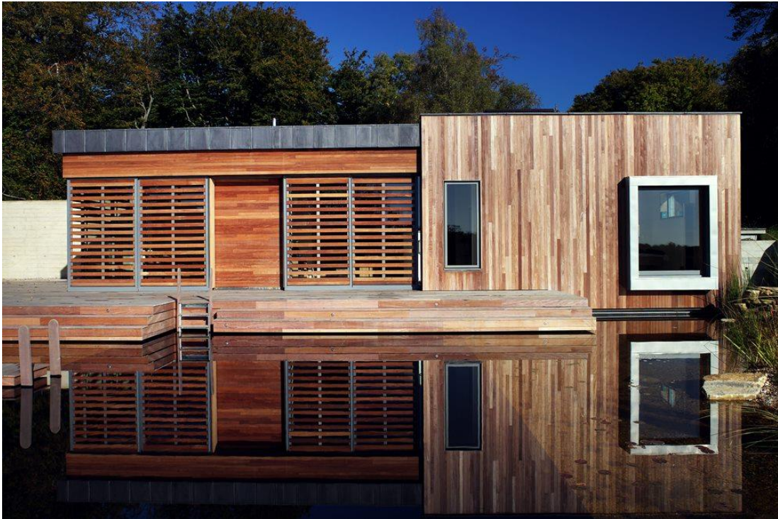
Effective use of louvres on this contemporary design to provide shading and reduce the impact of light spill from the large windows
