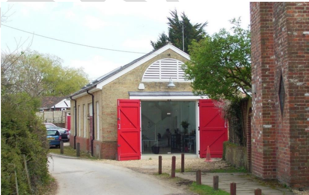
The successful conversion of the former Fire Station at Beaulieu into a design studio, which has retained the simple robust form and utilised existing openings
