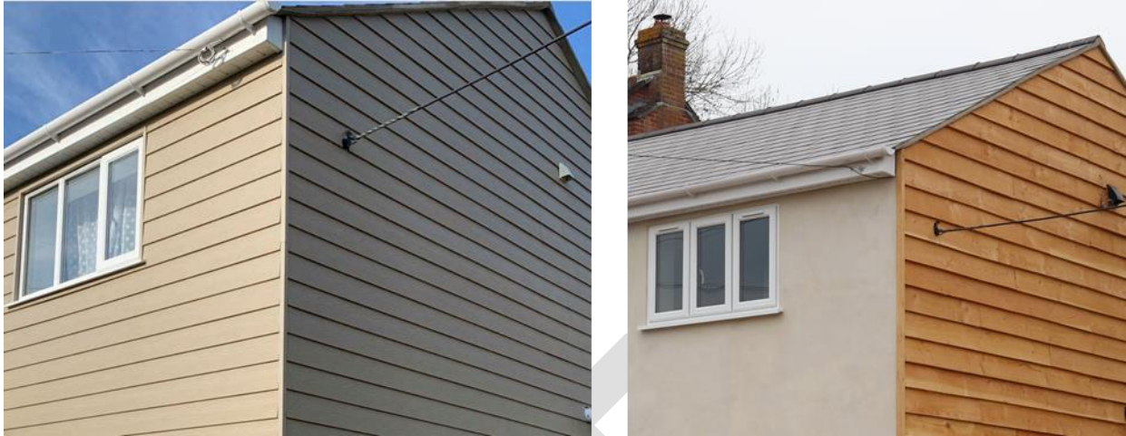
The same property clad with different materials: on the left clad with cedar cement boarding and on the right clad with natural timber which will weather to silver
