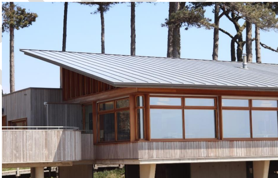
The metal standing seamed roof on the Lookout Café at Lepe Country Park
