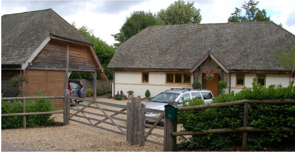
A shingle roof on a new build cottage in Burley
