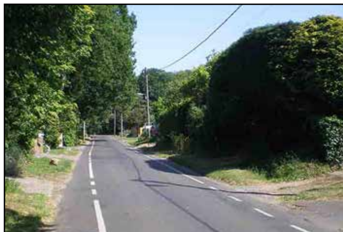
The narrow carriageway width on Wainsford Road
