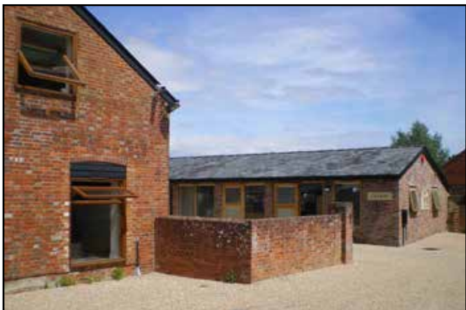
Office development at Efford Farm
