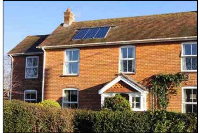
Use of solar thermal energy roof collectors in the Parish
