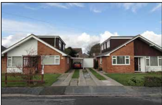
Impact of roof conversion at Pinewood Estate
