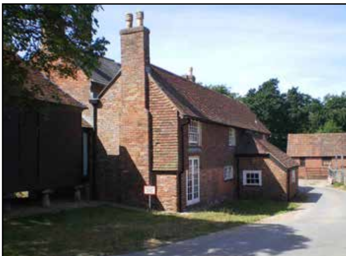
Listed buildings at Leagreen Farm
