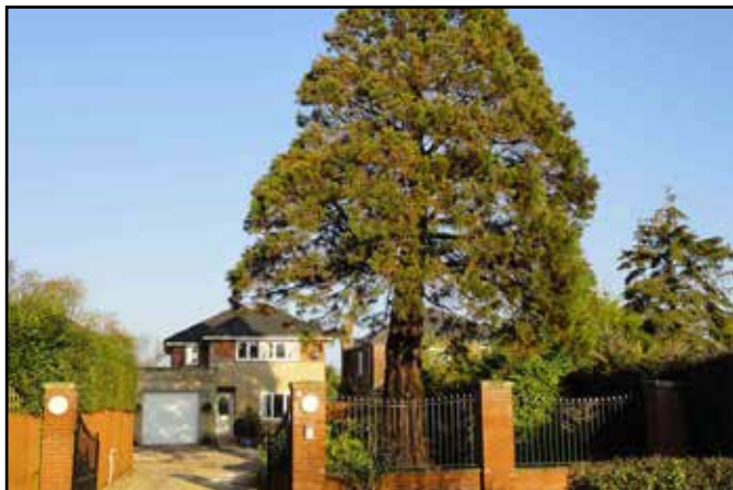
Gated development at Wellingtonia Gardens
