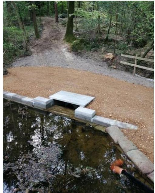
*The eel pass at Middle pond where adjustments and maintenance work has been carried out to keep the pond accessible to eels.*
