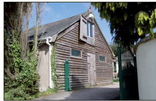
Timber render & usable roof space above
