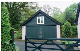
Separate garage with double pitched incorporating additional storage above
