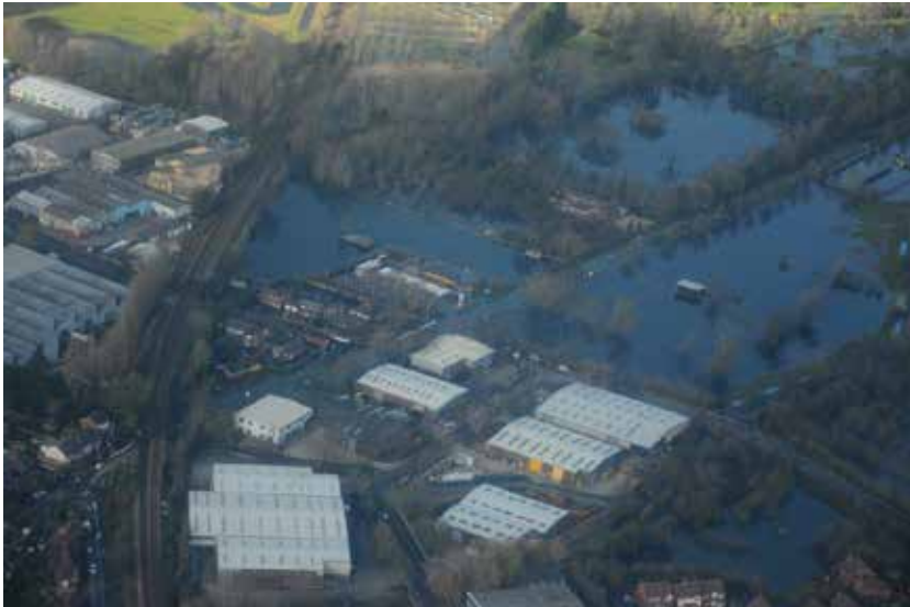
Flooding from the River Test in Romsey
