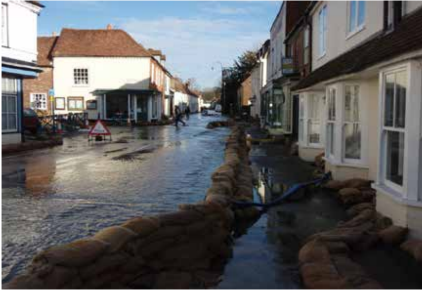
Groundwater flooding in Hambledon
