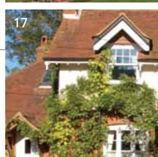
Photographs: 11, Decaying block-cut ridge; 12, Thatched roof with block-cut ridge; 13, Water reed for new thatch; 14, Re-thatching in water reed; 15, Thatcher's signature; 16 & 17, Plain clay tiles.
