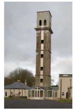
Trial tower c.1880 for ATT Peterson, early example of concrete construction
