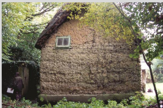
Figure 34 - Un-rendered and unprotected end elevation of clay cob building
