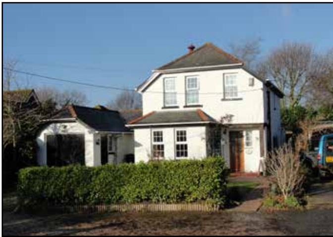
The Anchorage alongside Kings Farm is over 100 years old
