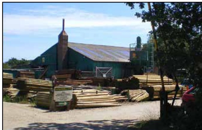
Construction & building materials business Crabswood Lane
