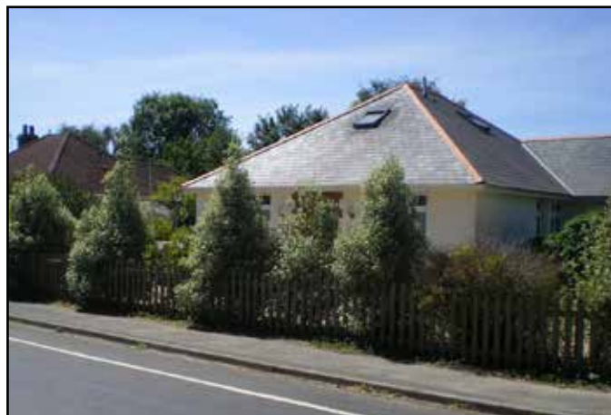
Refurbished bungalow in Wootton Road with slate roof
