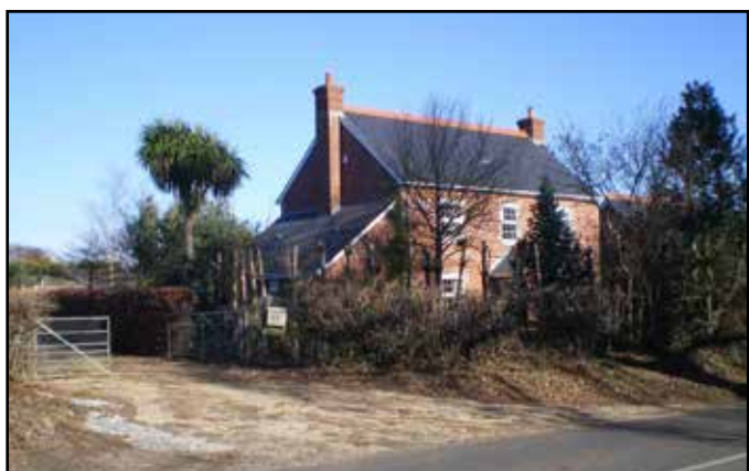
Brockhills Nursery with new build cottage c. 1997
