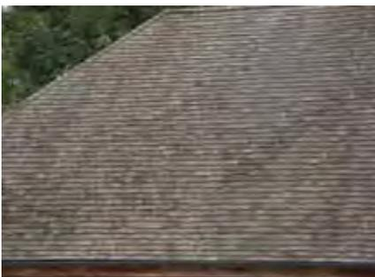
Oak shingles are not traditional to the area, but they are natural, with a small module and little wastage. They can be used on steep or shallow pitches and as a vertical cladding. They are small enough to create winding roofs and are lightweight when compared with tiles and slates. Avoid cedar because of acid run-off.
