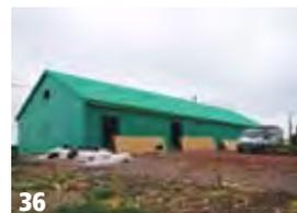
Insulated panels (SIPS) can receive traditional as well as contemporary claddings. They are an effective way of building quickly, while providing high levels of insulation. Shown here with a membrane, waiting to receive material.
