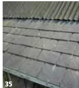
Recycled rubber slates can replicate the scale and tone of traditional slates. They may be appropriate where tone and module are the key qualities sought, in low key and non-traditional situations.
