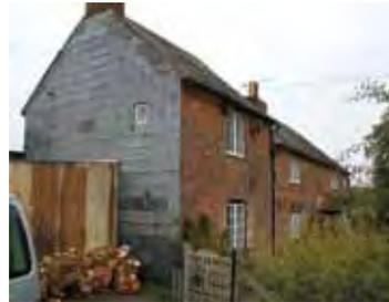
Slate is quite adaptable, shown here used vertically. It is also commonly used on shallow roofs.
