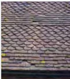
Clay tiles can have an antique finish, be natural terracotta allowed to weather, or a contrasting red, often used in vertical tile hanging. Avoid out of scale bulky interlocking tiles.
