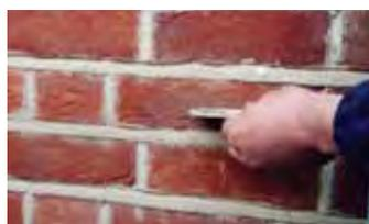
Brickwork, avoiding fatty joints to give brick a traditional look. Hampshire oranges and reds are common. A mix of the two will give a traditional dappled look. Silver grey mortar tone, avoiding bucket handle joints, will enhance appearance. Buff bricks are common, often used with slate. In some circumstances the use of lime mortar may be appropriate to give a traditional appearance.
