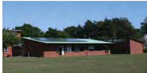
Flush solar panel on a monopitch roof.
