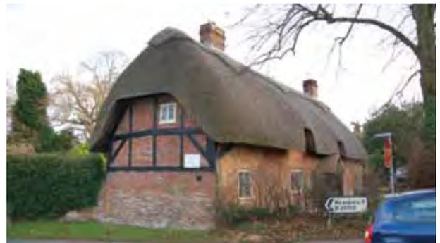
Thatch is appropriate for steeper roofs, avoiding fussy ridge lines and complicated roof forms and valleys. Roofs should use material prevalent to its locality.
