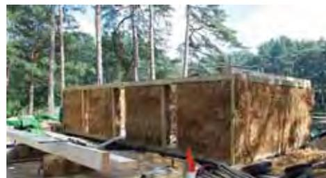
Straw bales used in conjunction with reinforcement to provide sturdy looking walls. They can be used to provide rounded corners and deep reveals. Elevations are often rendered. Roofs need pronounced overhangs to facilitate weathering.
