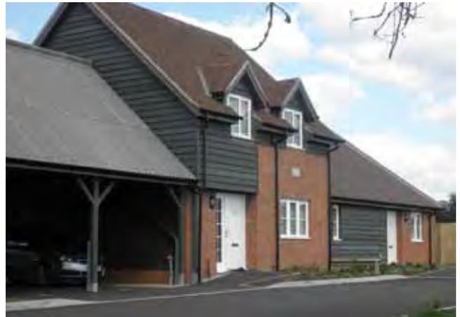
Rural tone: a combination of plum / orange bricks, tiled and corrugated roofing, and robust feather-edged cladding.
