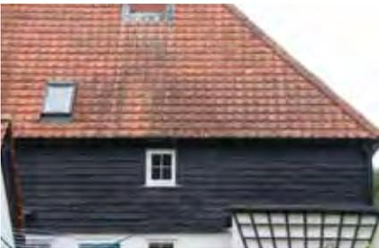
Modern small scale interlocking clay pantiles are available that reflect traditional characteristics. Pantiles are often seen on Arts and Crafts houses and farm buildings. New versions use modern interlocking techniques suitable for shallow and steeper roof pitches.
