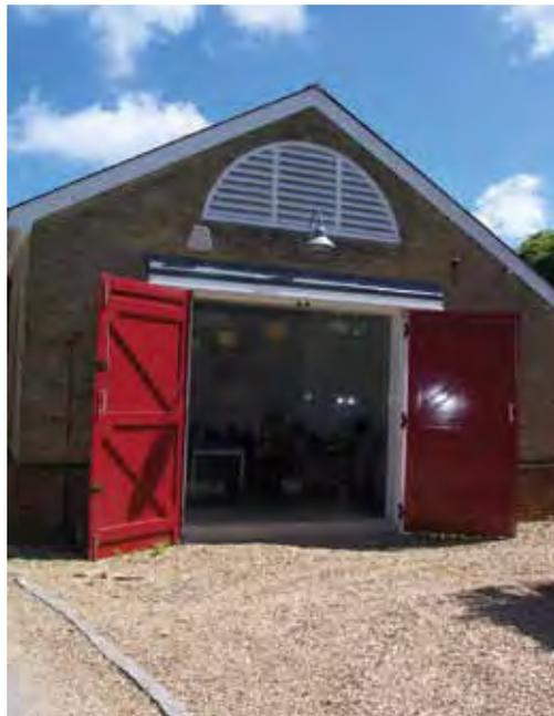
A former electric light station converted to office use. Its robust doors echo a past use and help reduce glazing impacts and heat build-up. Recessing glazing also reduces reflection.
