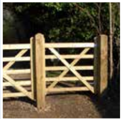
Timber five bar gate.
