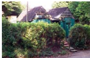
Shack built of makeshift materials
