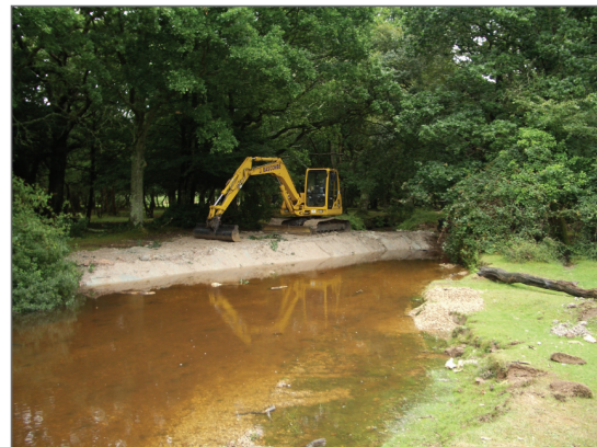
Constructing clay bund
