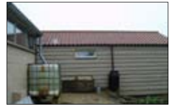
Opportunity to recycle water direct from roof
