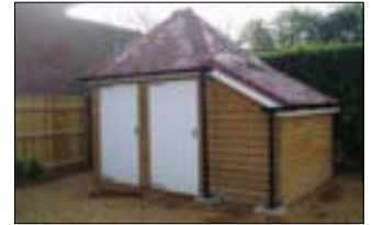
New build bin & bike store
