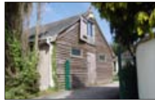
Timber render & usable roof space above
