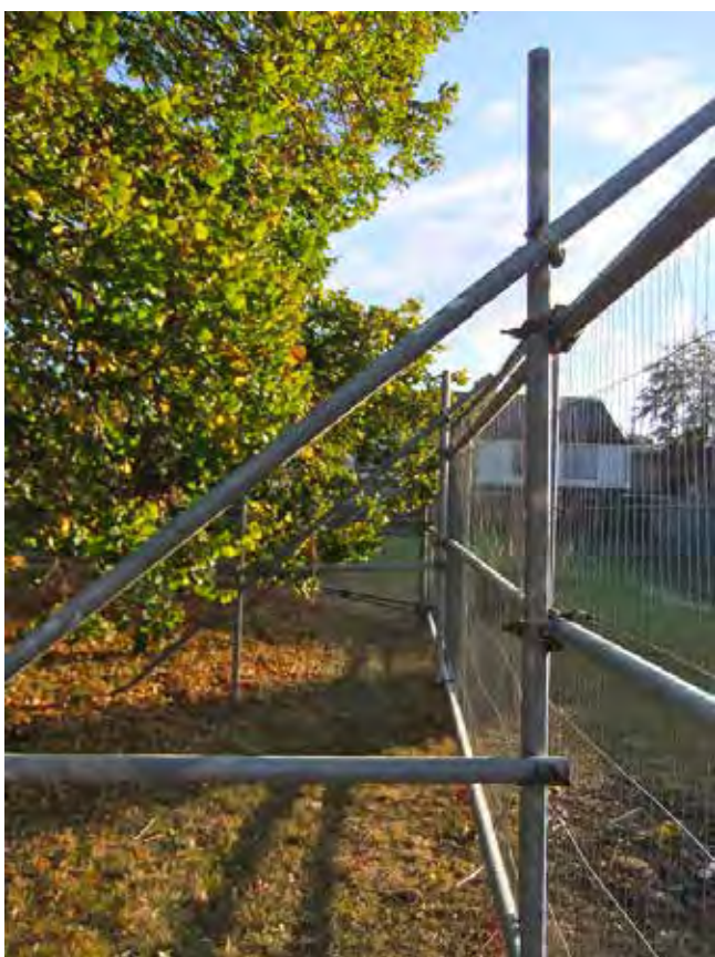
Typical scaffold braced protective fencing
