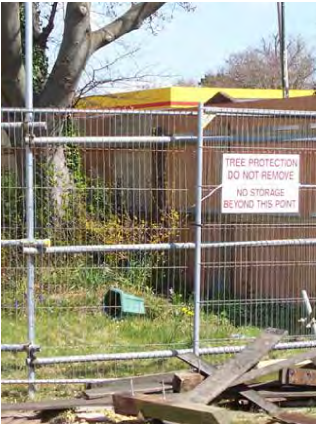
Signs can be useful to alert construction workers
