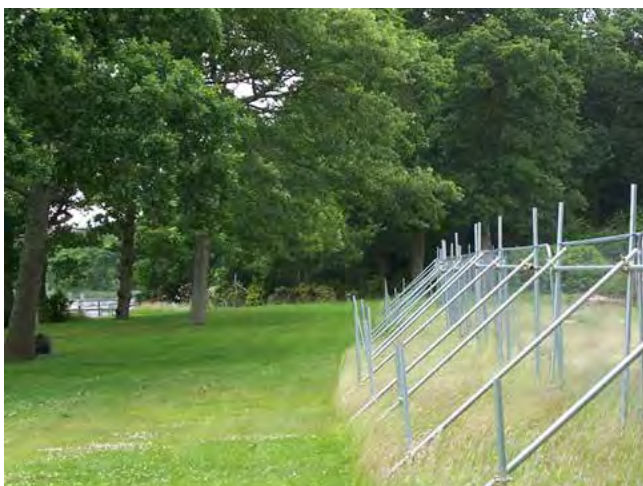
Fencing should be braced using a scaffold framework
