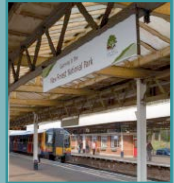
Brockenhurst train station
