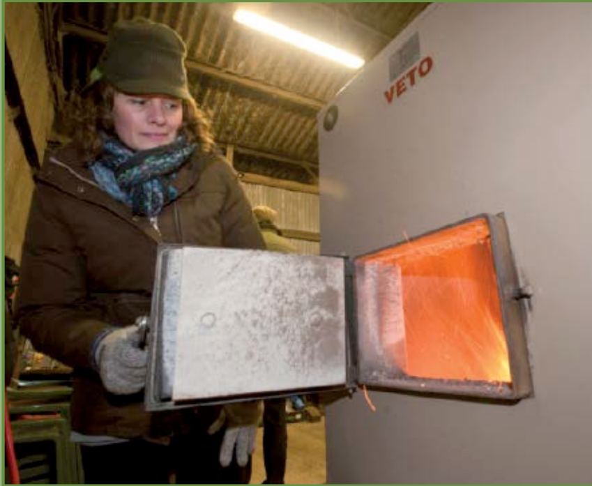
Wood fuel boiler at Ipley Manor
