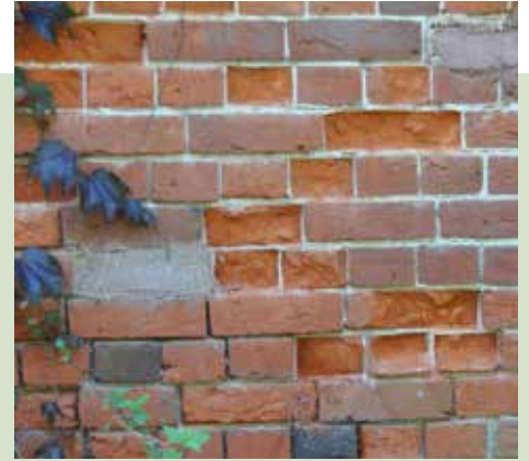
Example of damaged brickwork
