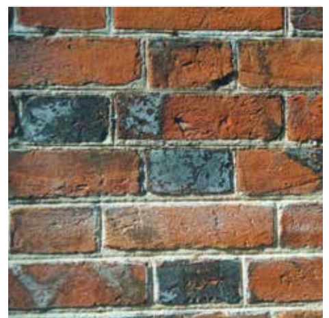
Fine brickwork with carefully finished jointed joints
