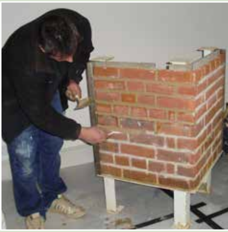
◀ Demonstration of re-pointing
