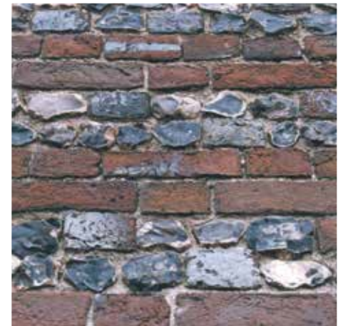
Brick and knapped flint detail
