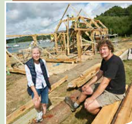
Building a Shipwrights School at Buckler's Hard
