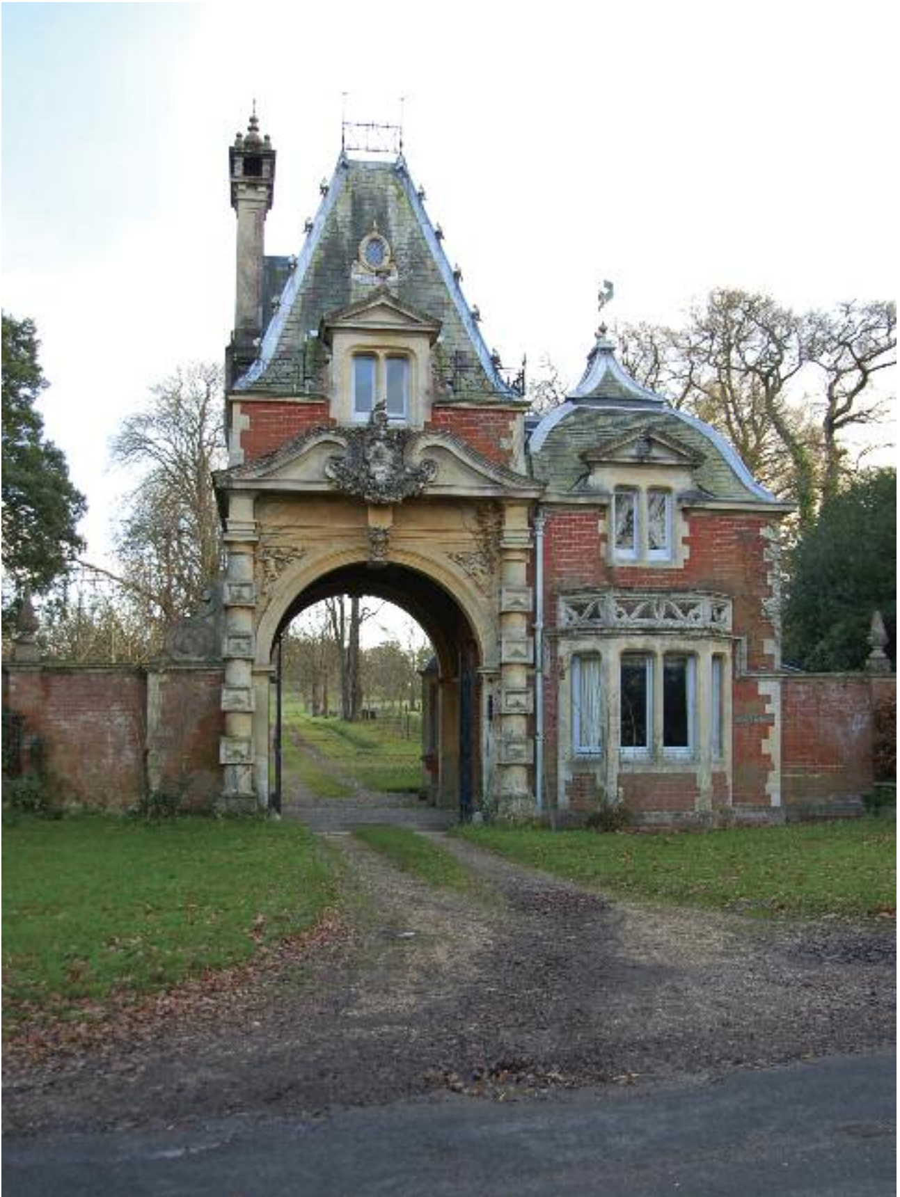
Lodge to Brockenhurst Manor
