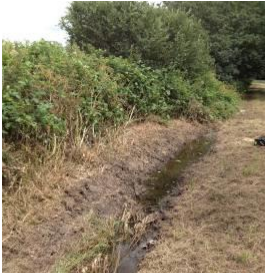
Grassy swales can be used to intercept runoff from roads but they become part of the problem if the vegetation is removed and bare soils exposed to erosion
