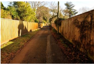
Close board fencing
