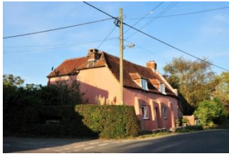
Unsightly power lines
