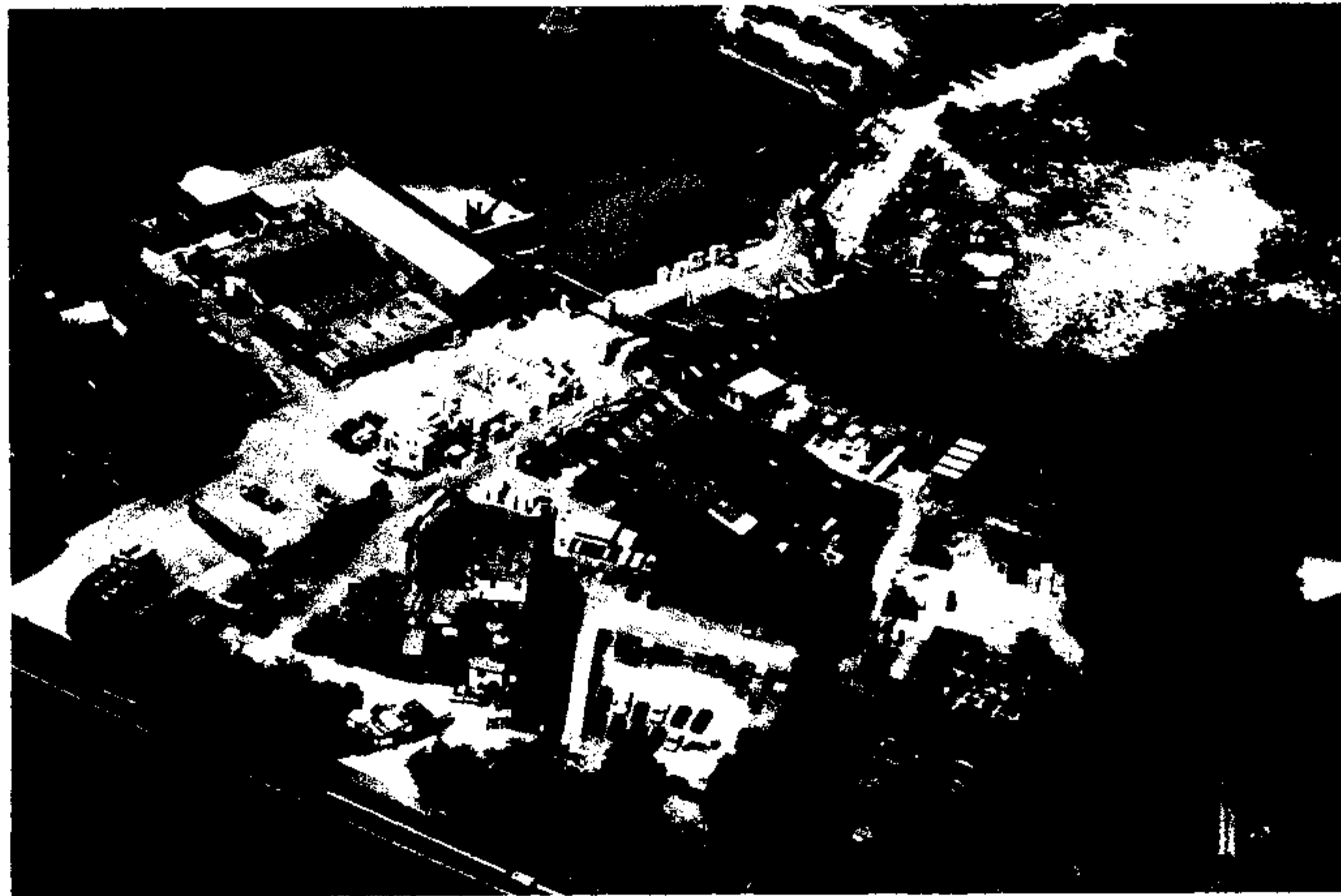
Photo 4 – Pre Fire Site
